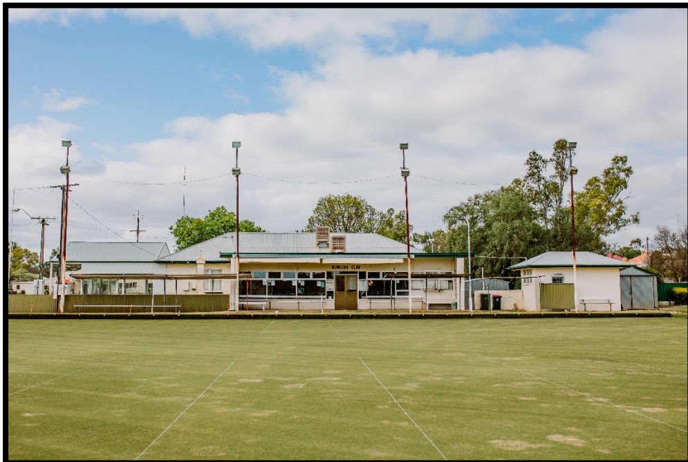
The Spalding Bowling Club were successful in obtaining $5,725 toward a solar energy installation
