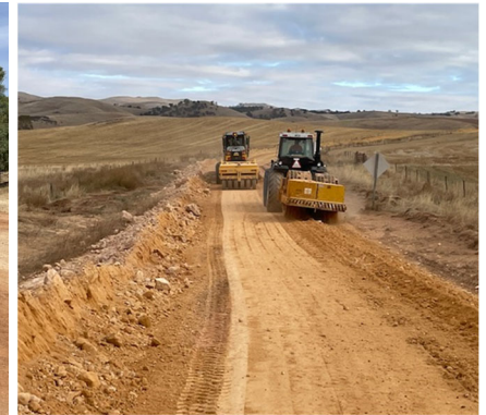
Resheeting Bundaleer Rd with raw material from Boultons Pit, Washpool
