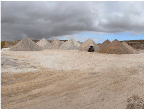
Crushed Rubble in Crawfords pit for re-sheeting of Cloverhill Abbeville Road near Georgetown.
