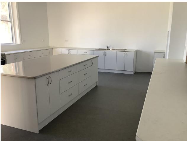
Completed works at the Jamestown Memorial Hall
