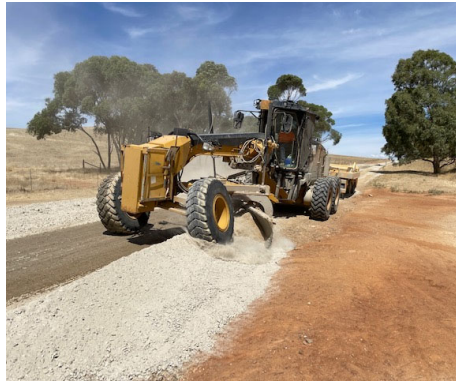
Resheeting Ward Hill Road with crushed material from Mundunney pit, Belalie East.
