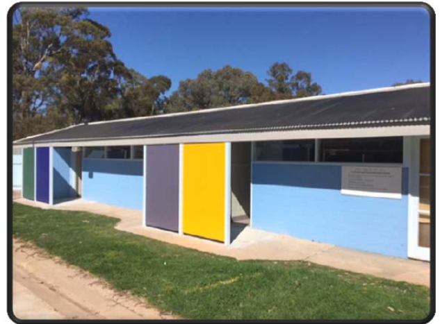
External view of changing room area.
