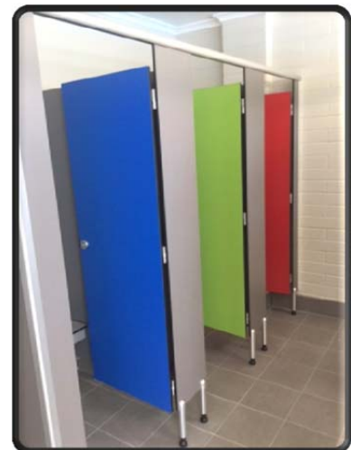
Newly established "changing" cubicles in female change room
