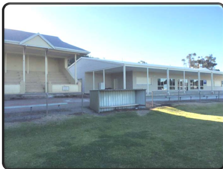
View from Oval of the newly constructed Sports Complex at Spalding Oval
