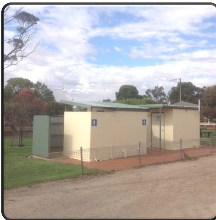
Georgetown Toilet facilities prior to demolition
