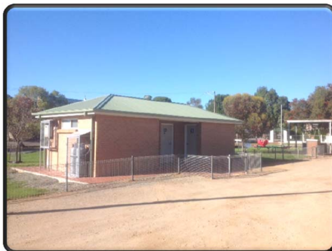
New toilet facilities at Georgetown Playground
