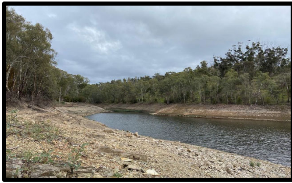
The Beetaloo Reservoir remains a key component in the Remarkable Southern Flinders Project
