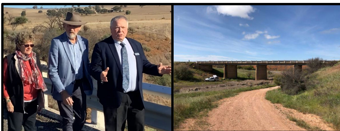
Council secured just over $2.9m in funding from the Federal Government’s Bridges Renewal Program to upgrade and widen the structure of the Pine Creek Bridge near Laura
