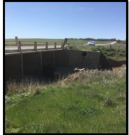
Andrews Bridge West 2020
