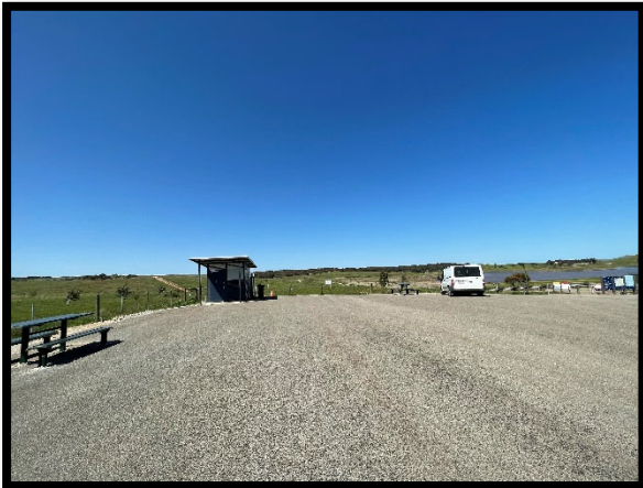
Bundaleer Reservoir carpark new seal 2021/22
