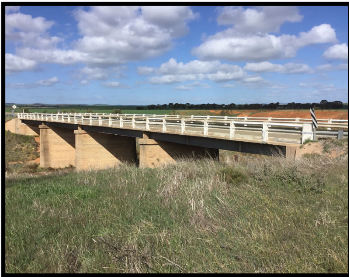
Pine Creek Bridge 2020
