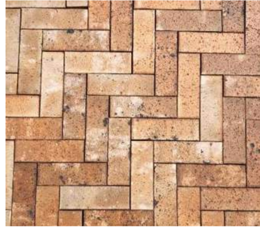
Brick unit paving Ayr Street footpaths
