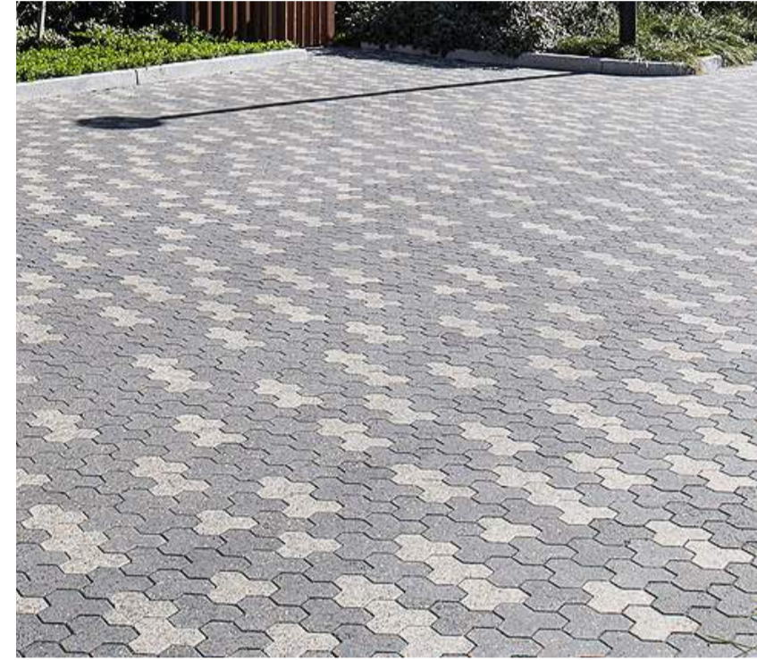
Concrete unit paver Raised crossover between Irvine Street & Ayr Street
